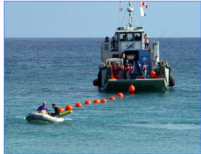
Laying Submarine Cable
