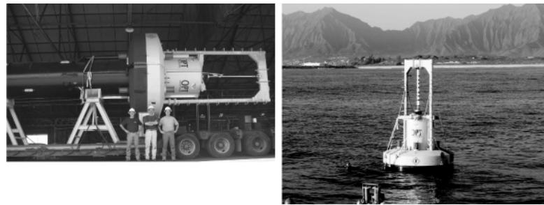
Our PowerBuoy system consists of a floating buoy-like device that is loosely moored to the seabed so that it can freely move up and down in response to the rising and falling of the waves, as well as a power take-off device, an electrical generator, a power electronics system and our control system, all of which are sealed in the unit.
