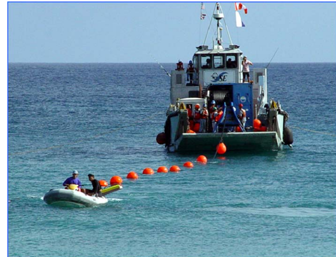
Laying Submarine Cable
